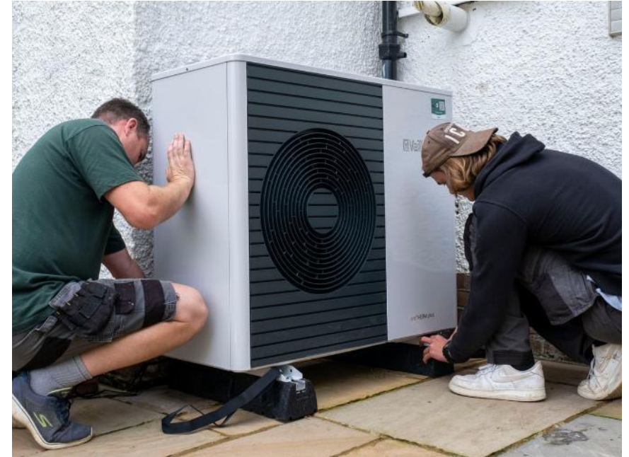
A High Temperature Heat Pump being installed.
